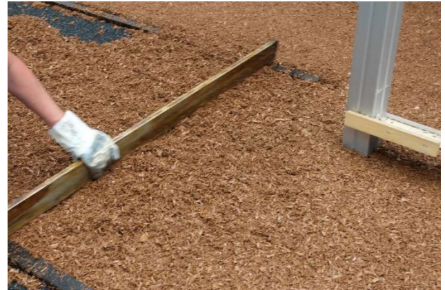
Levelling of the Melos EPDM mulch
